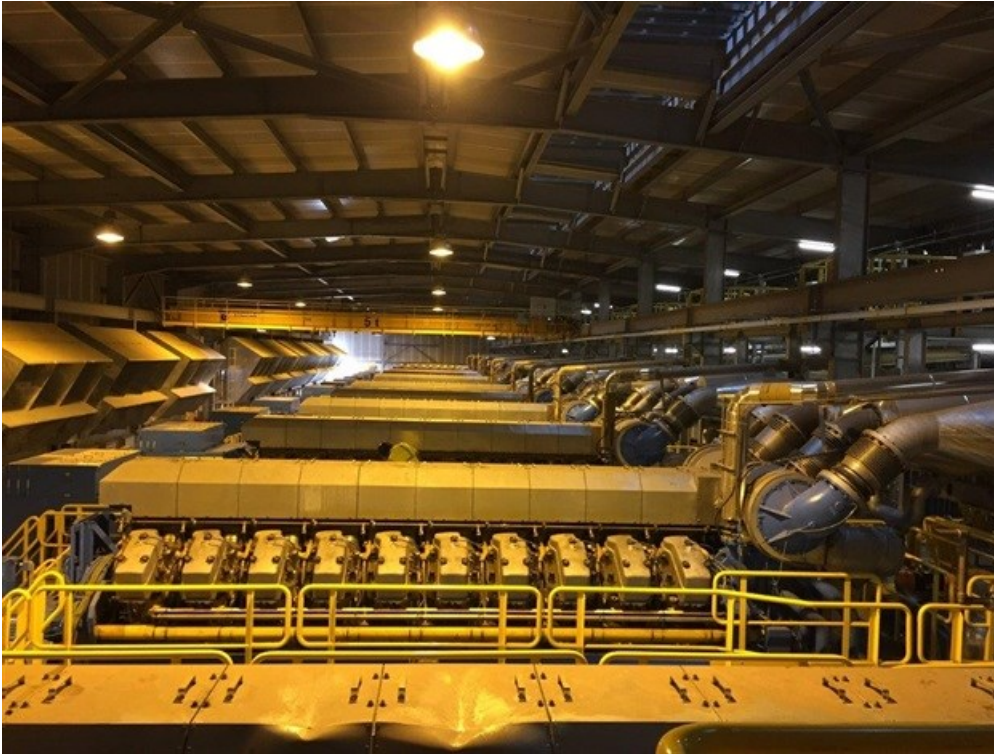
The Engine Hall of Gigawatt Mozambique's 120MW gas-fired power plant at Ressano Garcia showing the 13 Rolls Royce Engines.
