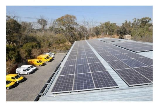
The Bryanston facility has a 10,000l rainwater harvesting system and rooftop solar energy generation plant, lowering the building's carbon footprint and reducing energy consumption by 55%. The reduced energy consumption is partly due to a 34kW solar photovoltaic system that reduces the demand for grid power by at least 25%.
