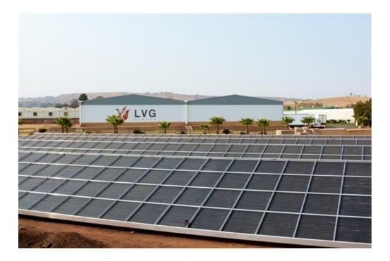
It is anticipated that 80% of LVG Plants' greenhouse heating will now be powered through their solar collector field with only 20% being generated from coal. Apart from greatly reducing their carbon footprint due to far less coal emissions, LVG will also reap significant energy cost-savings and they expect their investment in the solar infrastructure to break even within five years.
